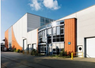
nora systems_Headquarter Weinheim A
