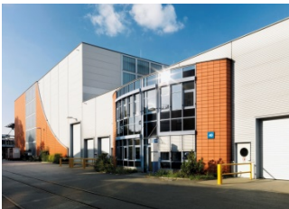
nora systems_Headquarter Weinheim A
